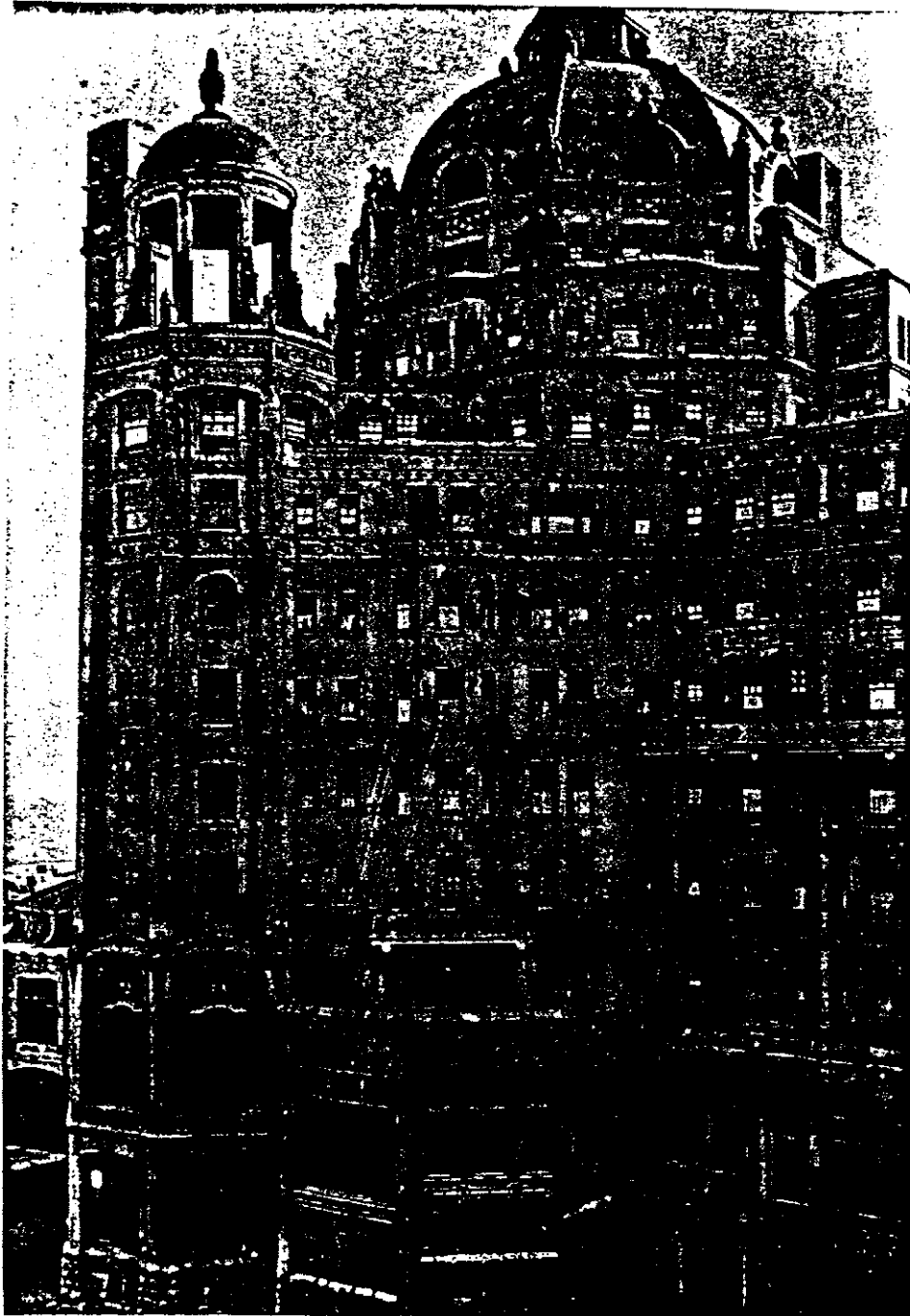
Hotel Blenheim, Atlantic City. (Price archive, collection George E. Thomas: hotel at completion, 1906).
